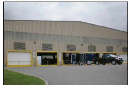
Photo 9-11: Waste management facility with receiving doors for self-haul traffic that are completely separated from the doors used by larger waste collection vehicles © CH2M HILL
