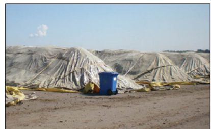
Photo 5-15: Covered, positively aerated composting system © CH2M HILL
