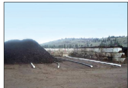
Photo 5-13: Typical ASP system with aboveground piping; block walls separate batches to better utilize available space © CH2M HILL
