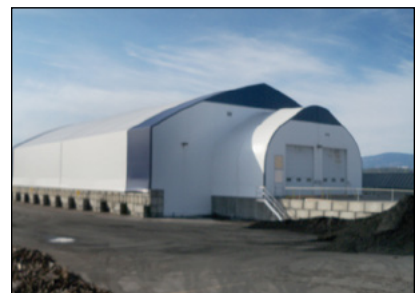
Photo 10-2: Fabric-style receiving building © CH2M HILL
