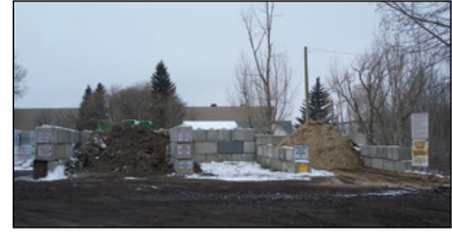
Photo 12-2: Bunker: ecology-blocks used at an L&YW drop-off depot © CH2M HILL
