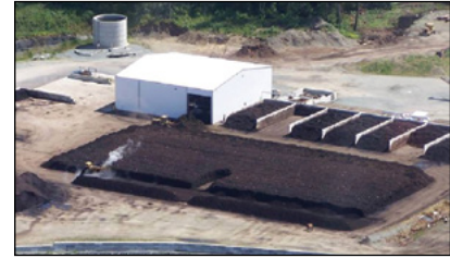
Photo 5-10: A mass bed system in the process of being turned; note turner location at bottom left of the pile and aisle created behind the turner © Lenz Enterprise Inc.
