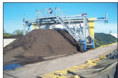
Photo 5-16: Mobile unit used to place and remove covers © CH2M HILL
