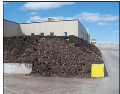
Photo 14-6: Unenclosed biofilter at a composting facility © CH2M HILL
