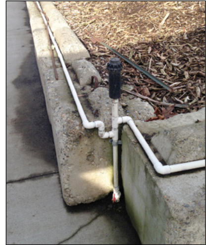
Photo 14-7: Water can be added to biofilter media using sprinklers, but care must be taken not to overwater the biofilter media © CH2M HILL
