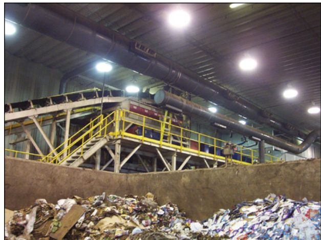
Photo 3-1: Both manual and mechanical methods are used for feedstock inspection and preparation © Scott Gamble
