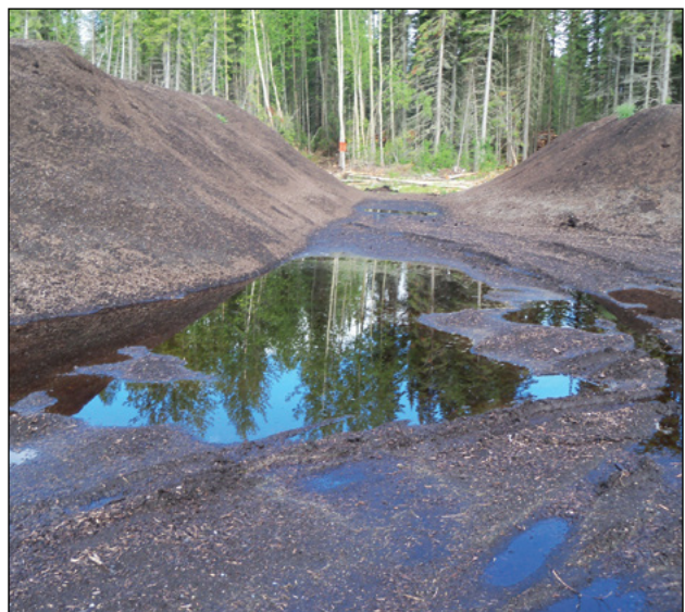
Photo 10-6: Water ponding in a compost facility's product storage area can affect access and lead to odours © CH2M HILL
