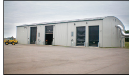
Photo 10-3: Engineered steel frame receiving building © CH2M HILL
