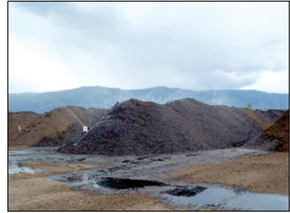
Photo 5-4: Water can be added to windrows and stockpiles using sprinklers © CH2M HILL
